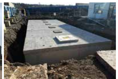
Underground water tanks
