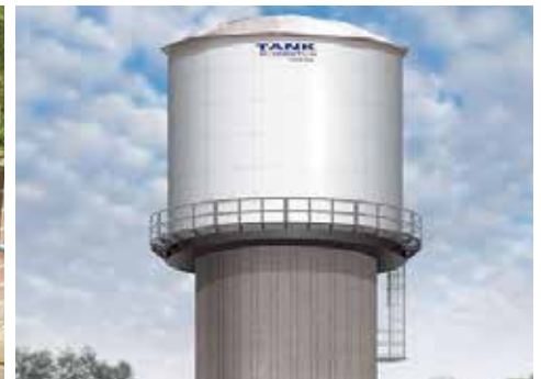
Overhead water tanks
