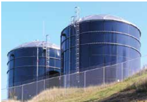
Commercial water tanks
