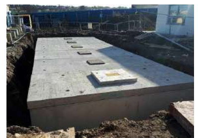
Underground water tanks
