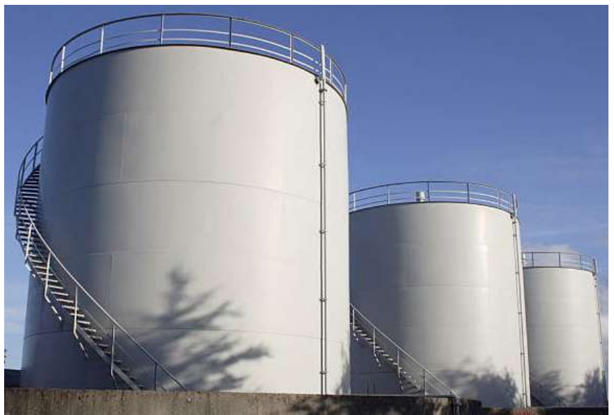
Industrial water tanks
