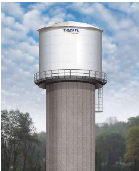
Overhead water tanks
